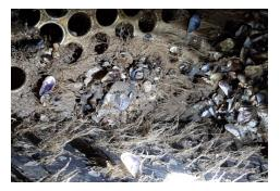
Image 1: Macrofouling of condenser caused by mussels and debris
