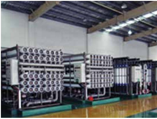
Figure 1 and 2 - UF + RO wastewater recycling system
